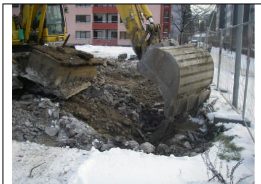
Schaktning massor under spolplatta
